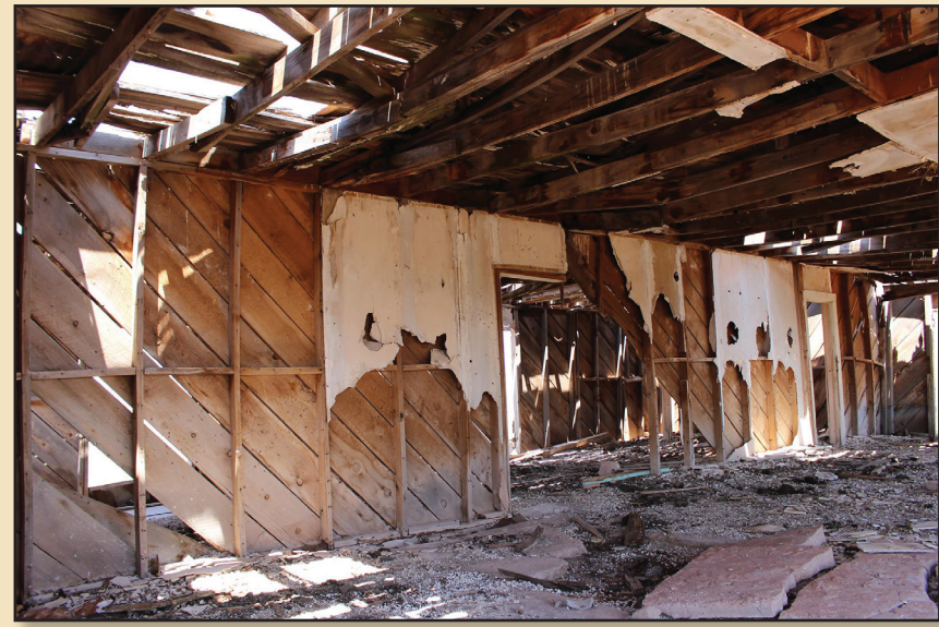
Cattle had completely destroyed the wall beneath the west front window.
