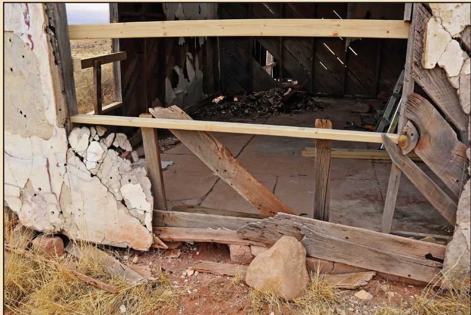
Cattle had completely destroyed the wall beneath the west front window.
